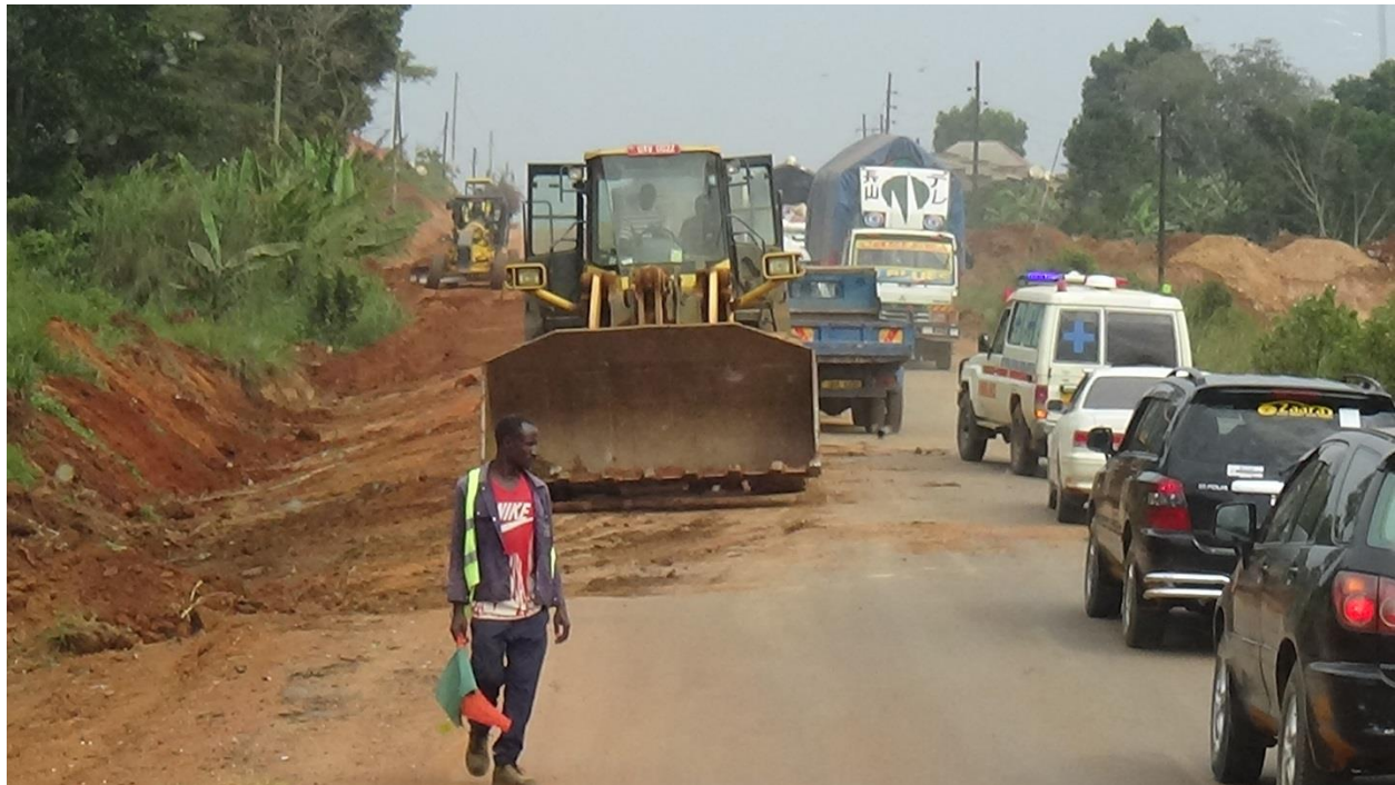
Figure 5: above showing a traffic control person guiding traffic at a location with active project works.
